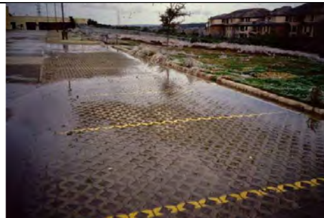
Water standing on the parking surface 48 to 72 hours after a storm is an indication of clogging. Snow piles at the edge of the photo point to possible clogging from winter sanding or plowing.
